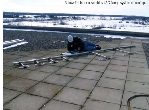
Below: Engineer assembles JAG flange system on rooftop.
